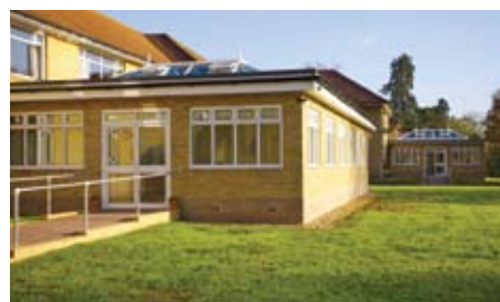
Ground floor extensions to Albert and Elizabeth houses
